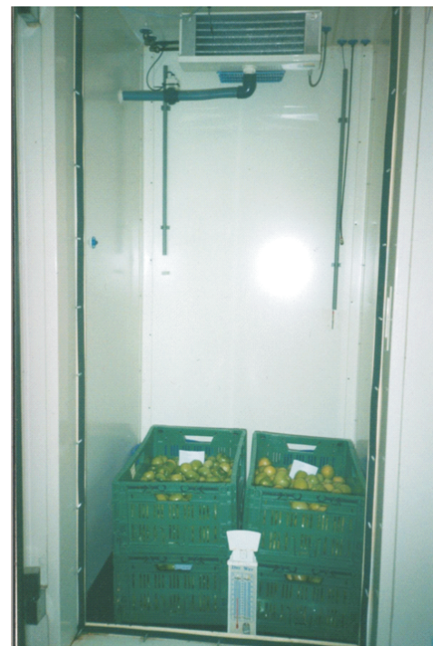
Figure 2. Controlled Atmosphere storage chamber
